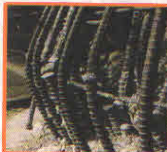
Damage due to insufficient gas pressure welded splices. Longitudinal reinforcement broke at pressure welding portion in Kobe earthquake.
