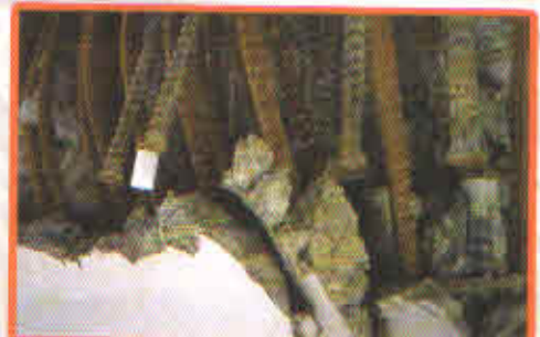
A fairly common feature of bridge column failure was the popping of gas pressure welded splices, which represent fairly common Japanese practice. These splices failed frequently in older buildings, and occasionally in new construction.
