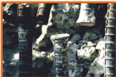
Failed welds at splices of longitudinal reinforcement in a column supporting the Hanshin Expressway (at the 500-meter-long failed section). These gas fusion welds are 1960's technology and are not common today in the United States.
